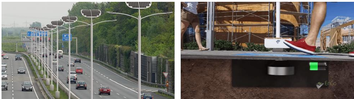
Figure 18: Self-powered smart street lights from solar energy (left), resp. solar and vibration energy (right) [39]
