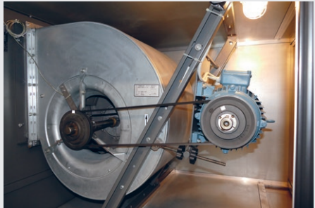
Fan-MDU (from left to right): fan, mechanical equipment (belt), motor (Source: Impact Energy, 2016)
